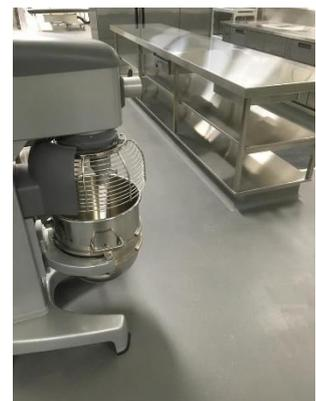
Dry goods packaging, clean rooms and amenities areas are typically suitable for epoxy applications. In fact, you will find that epoxy coatings may be suitable in most areas where light to medium duty requirements are present.
